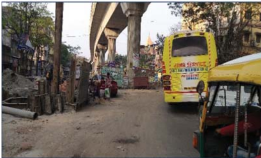
Plate 3: Road diversion at Silpara
