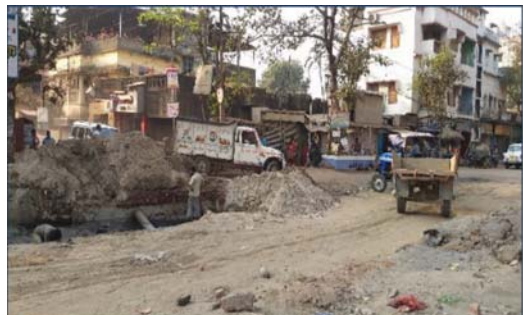
Plate 4: Excavation at DH Road for Metro construction
