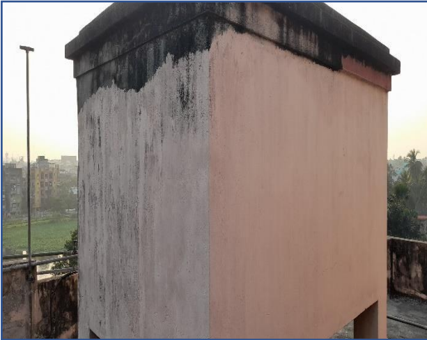
WATER RESERVOIR IN ROOF TOP OF THE COLLEGE
